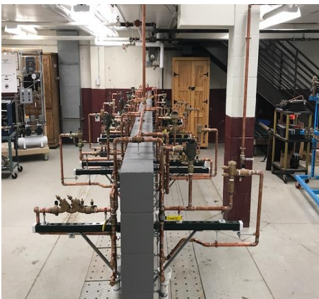
New Plumbing shop at St. Paul College!
